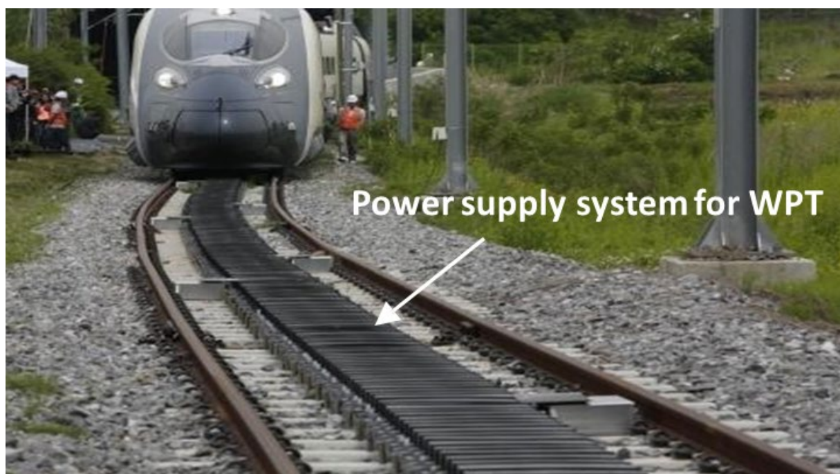
Figure 18 – 1 MW DWPT for next generation HS train
